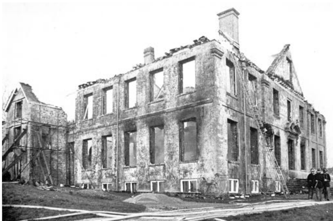
The roofless house after the fire in November 1967. Author's collection
