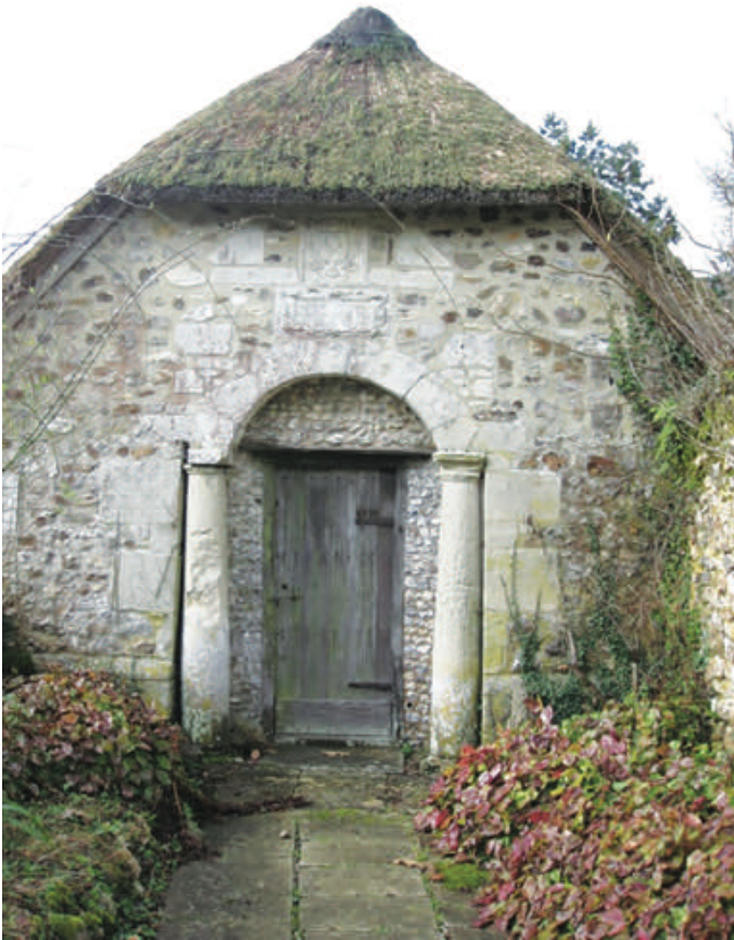
Northeast aspect of the garden building at Sand, showing the Tuscan columns, heraldic and macaronic inscriptions. Author's photograph 2012
