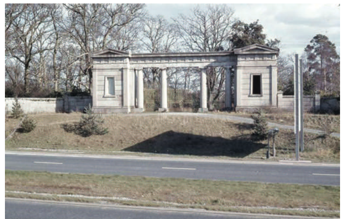
Granite Lodge entrance (1833) Historic England Grade II* and on 'At Risk' register
