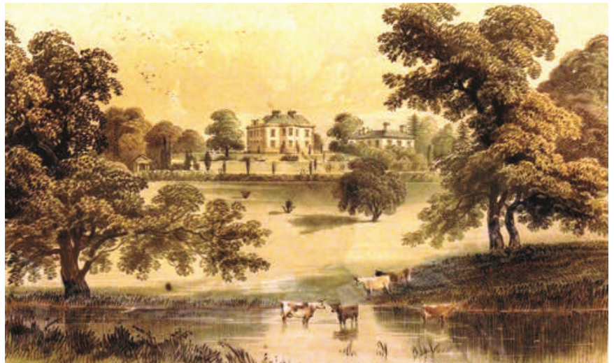
1855 Engraving by Daimond for twelfth Duke of Somerset showing improvements including Ionic temple, terraces and new servants' wing
