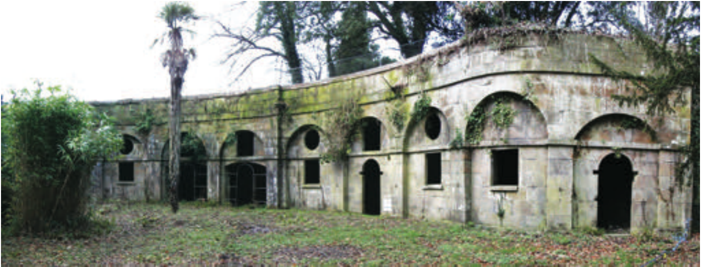
Templer's original stable block (Grade II*) 'The most significant building on the estate' (Historic England) and on 'At Risk' register
