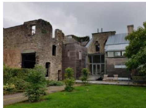
North-west façade of house with recent remodelling by current owners.
