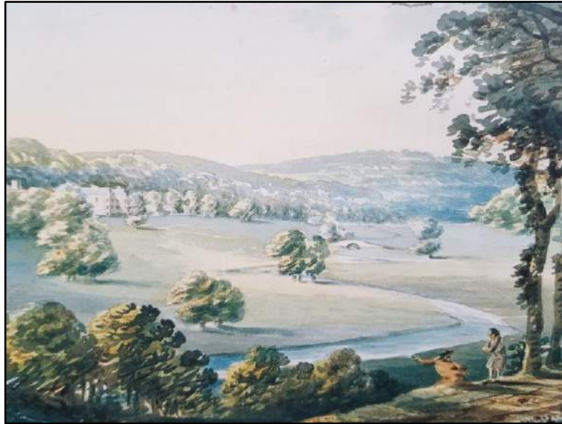
Figure 1. North East View of Eggesford - Old Eggesford House and Rosepool Bridge, DHC 564M/F11/99.
