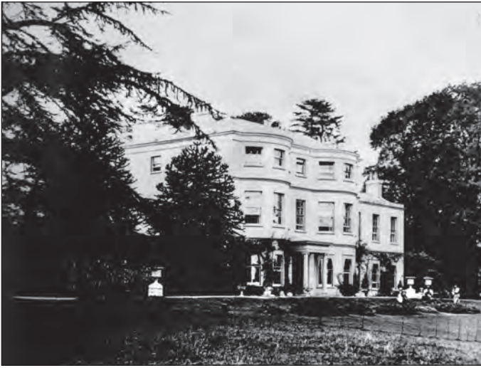
Figure 6. Cowley Place, 1875, John Hare, The History of Cowley Place , Plate 3.
